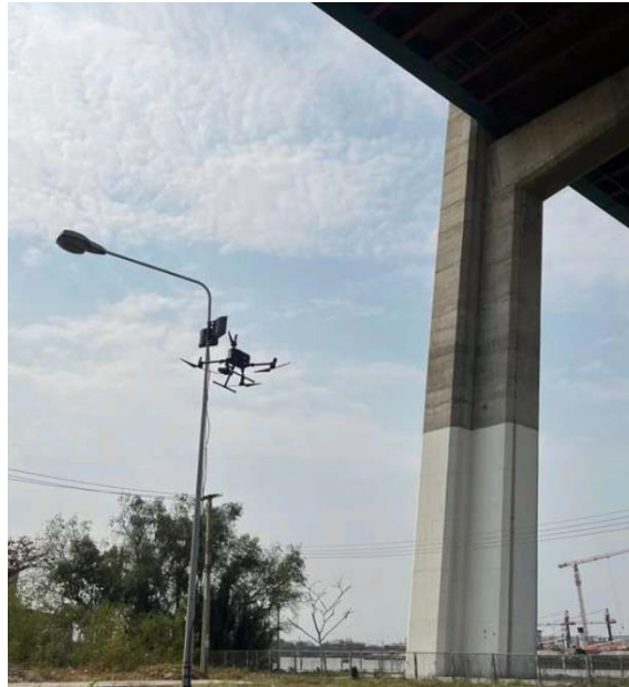
Figure 1 Field deployment and remote data acquisition utilizing the multi-payload UAV platform at the Kanchanapisek Bridge.
